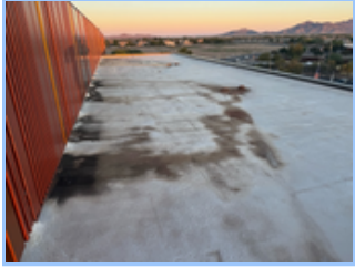
Foam Roof pic 001.jpeg
