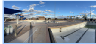
Rec pool plaster
