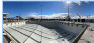
Comp pool plaster
